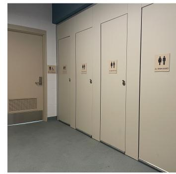
The floor isn't level across the whole building due to the drainage system, which meant special attention had to be paid to the bottom of the partitions to make them truly floor-to-ceiling for optimal privacy. Customizations included installing trim to close gaps between the partitions and ceiling and adding a sweep to the bottom of each door to eliminate any visible openings due to the uneven floor. Throughout the installation, the team tested for potential sightlines by measuring gaps on-site.
