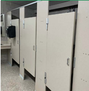
VIEW OF HINY HIDERS PARTITIONS AT HAMMOND MILL CAMP
