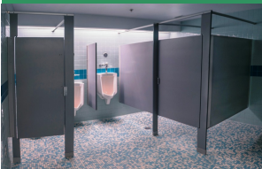
San Diego Pier Hiny Hiders Bathroom Partitions
